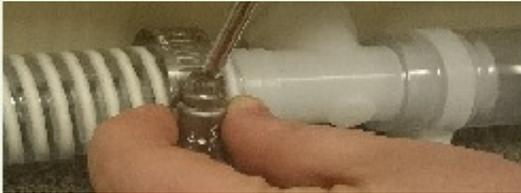
A good quality 1 1/2 cm interior diameter hose and a 1 1/2 cm stainless steel hose clamp will be required (can be purchased at a local building supply store). Carefully push the drain hose over the barbed end of the drain assembly so that the drain hose will overlap the drain assembly by 1 1/2 cm and tighten the hose clamp to secure.
