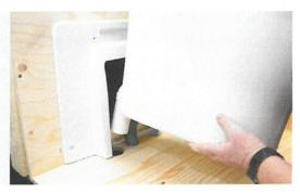
**8.** Put the bottom part into place against the floor and wall plate. Screw the bottom part into the wall with the two screws.
