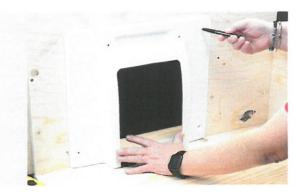
2. Measure or use the included template and mark the holes for the ventilation-pipe and urine drain (depending on model).
