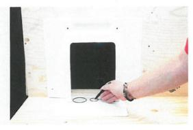
**3.** Drill holes in the floor for ventilation pipe 60 mm and possibly urine drain 40 mm.
